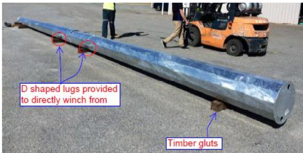
Figure1: Pole sections loosely assembled with forklift ready for joint assembly.
