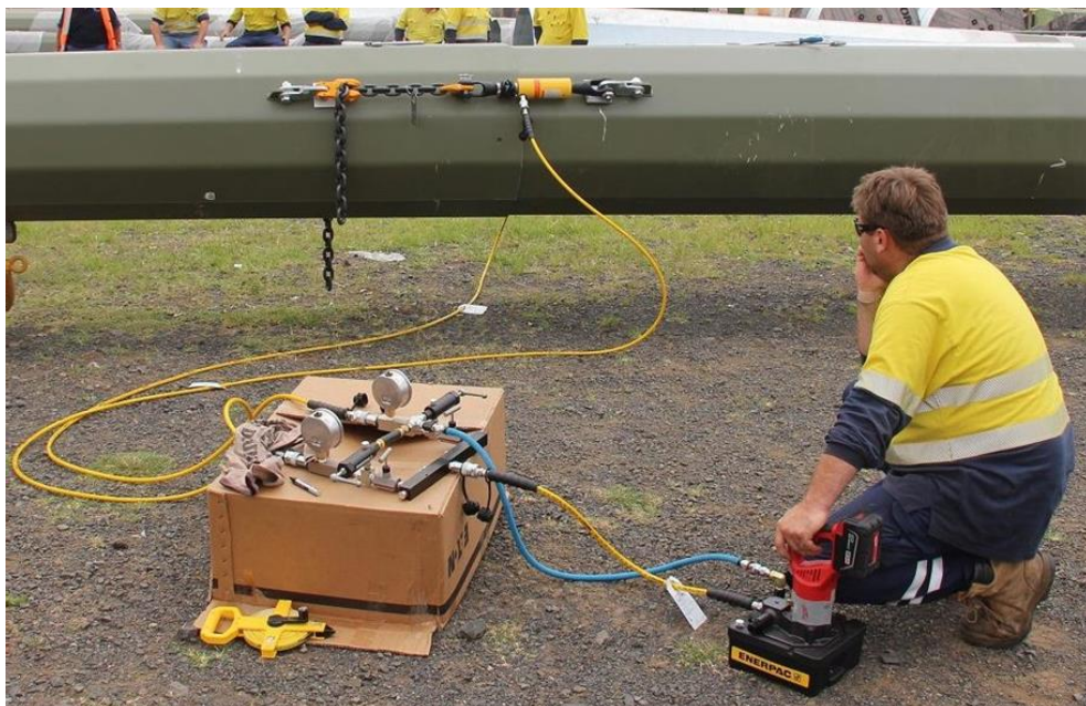
Figure 2: Joint assembly equipment utilising D type jacking brackets.
